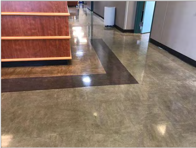
Accessible interior path (ramp/lift)
