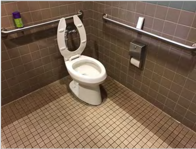
Toilet stall overview
