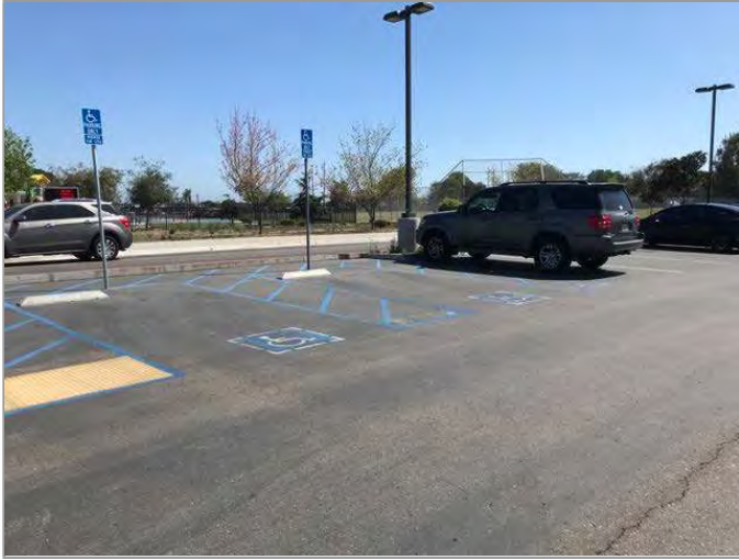
Overview of accessible parking area
