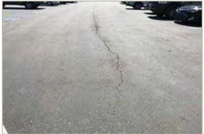
3 – ASPHALT CRACK
