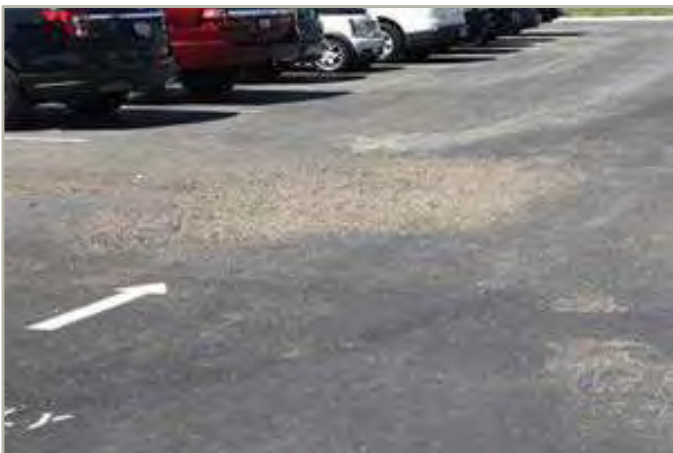
5 – ASPHALT DETERIORATION
