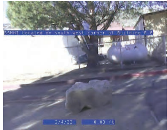
CCTV Entry Point Overall
