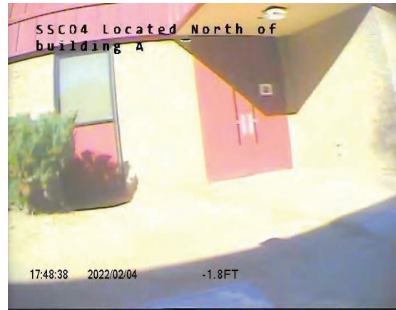
CCTV Entry Point Overall
