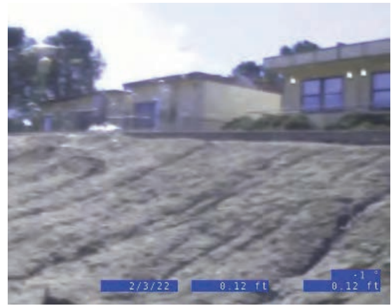
CCTV Entry Point Overall
