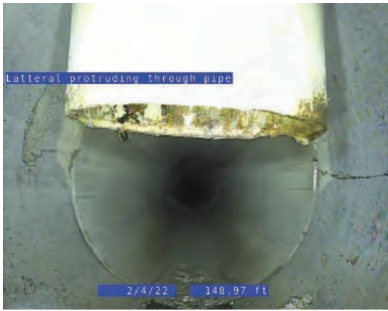
Lateral from Above at 148.97 ft.
