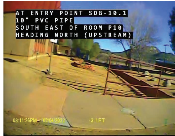
CCTV Entry Point Overall
