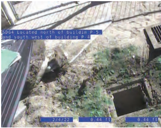
CCTV Entry Point Overview
