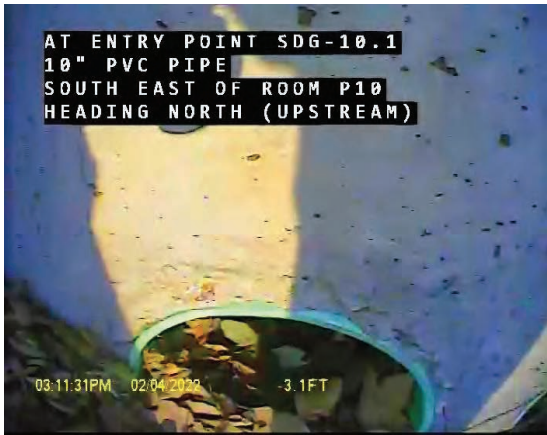
CCTV Entry Point Overview
