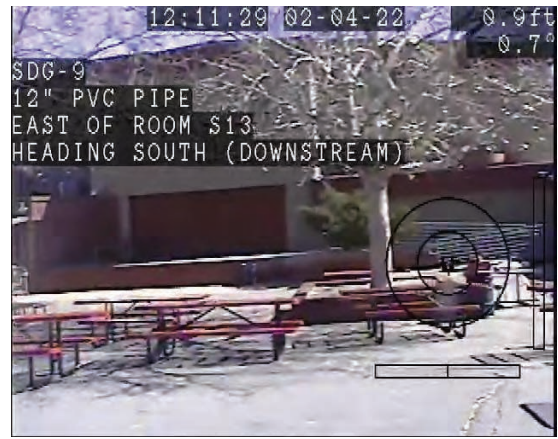
CCTV Entry Point Overall
