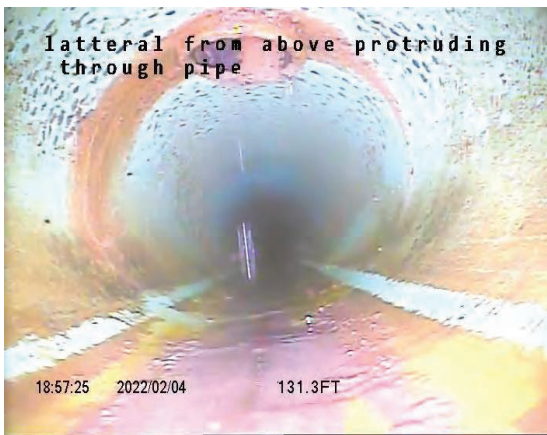
Lateral from Above at 131.30 ft.
