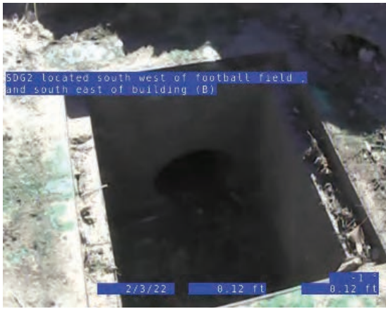
CCTV Entry Point Overview
