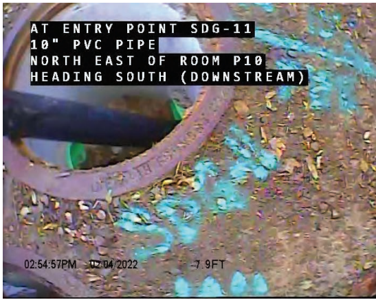
CCTV Entry Point Overview
