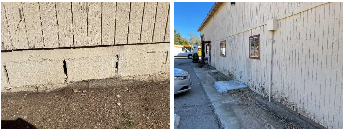
Grounds Shop Building Exterior –
