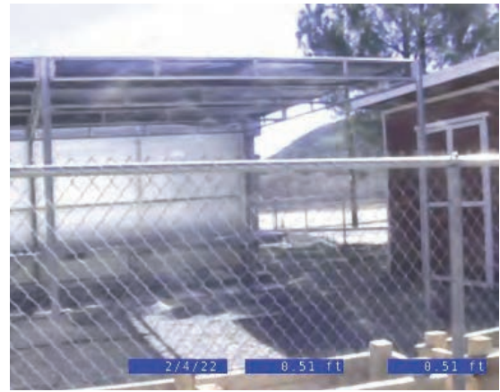
CCTV Entry Point Overall
