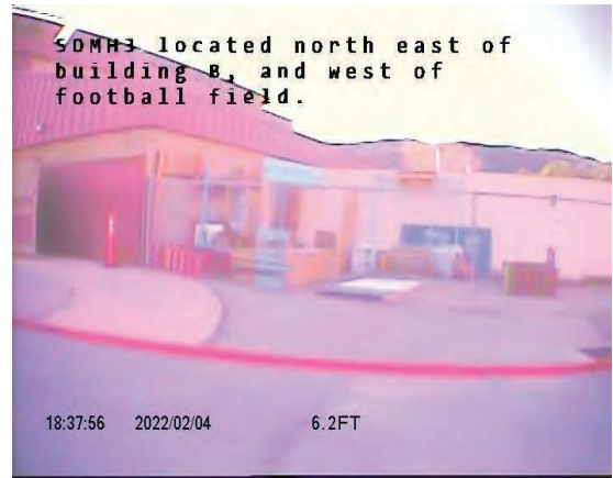
CCTV Entry Point Overall
