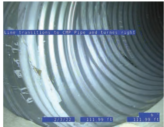
Pipe Changes to CMP at 111.99 ft.
