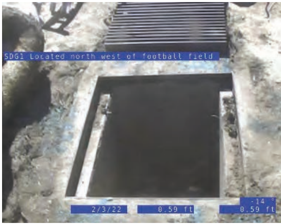
CCTV Entry Point Overview
