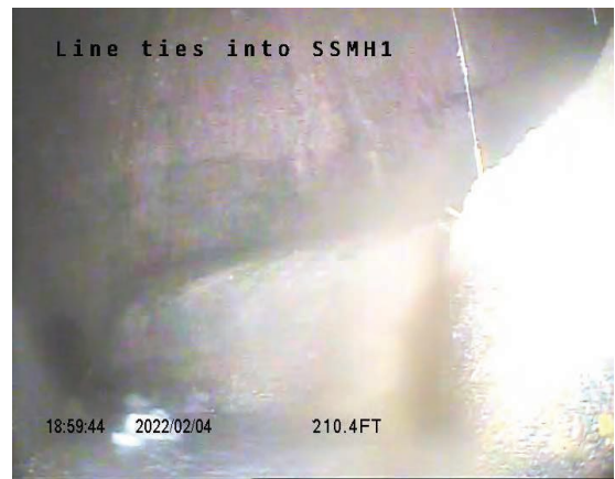
Ties Into SSMH-1 End of Run at 210.40 ft.
