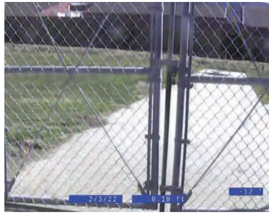
CCTV Entry Point Overall
