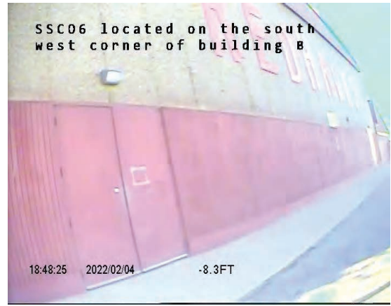
CCTV Entry Point Overall
