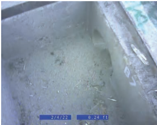
CCTV Entry Point Overview
