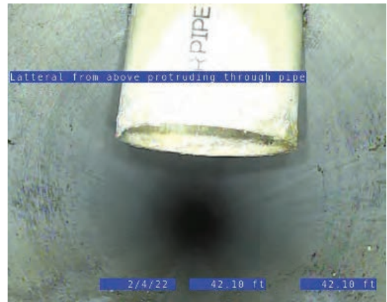
Lateral from Above at 42.10 ft.
