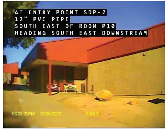
CCTV Entry Point Overall
