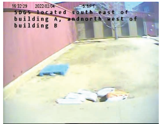
CCTV Entry Point Overall
