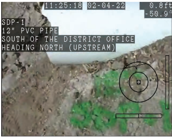
CCTV Entry Point Overview
