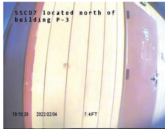
CCTV Entry Point Overall
