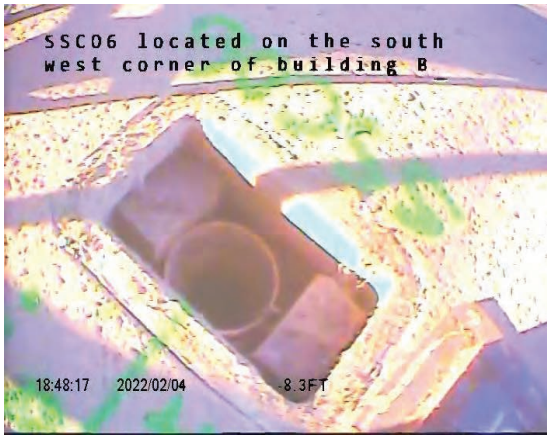
CCTV Entry Point Overview
