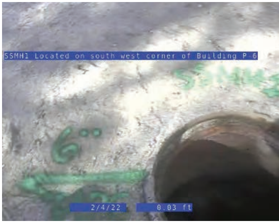
CCTV Entry Point Overview
