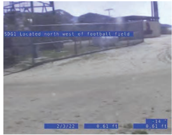
CCTV Entry Point Overall
