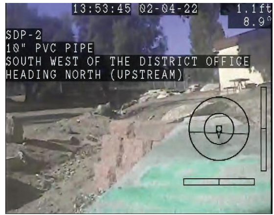
CCTV Entry Point Overall
