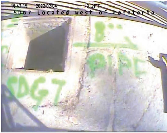
CCTV Entry Point Overview
