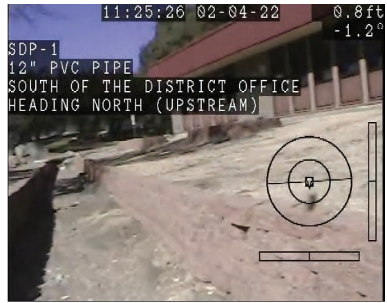
CCTV Entry Point Overall
