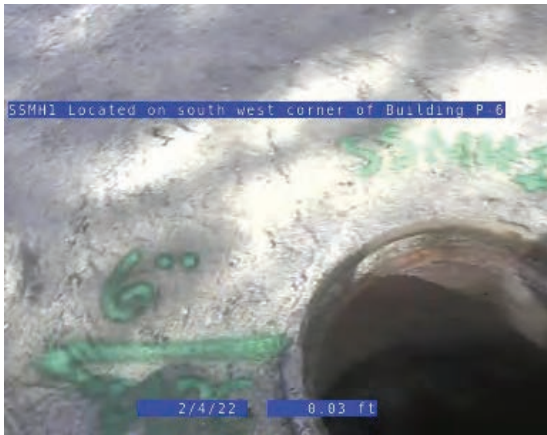
CCTV Entry Point Overview
