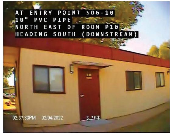
CCTV Entry Point Overall
