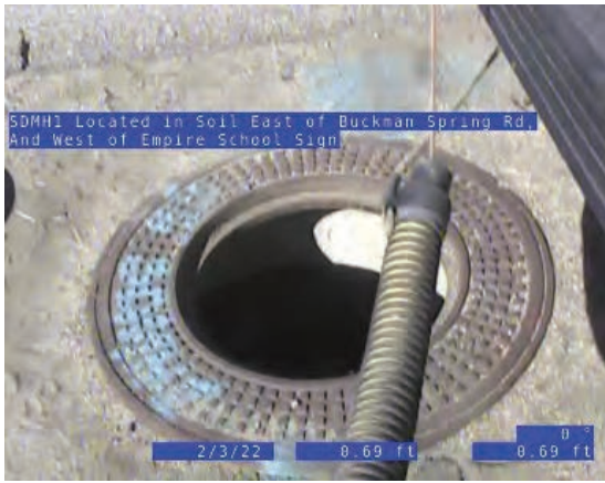
CCTV Entry Point Overview
