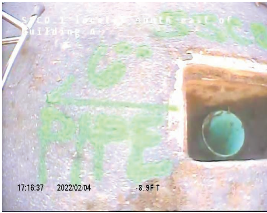
CCTV Entry Point Overview
