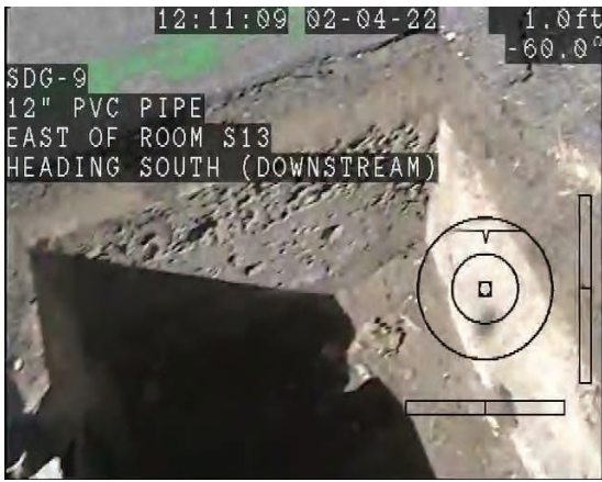
CCTV Entry Point Overview
