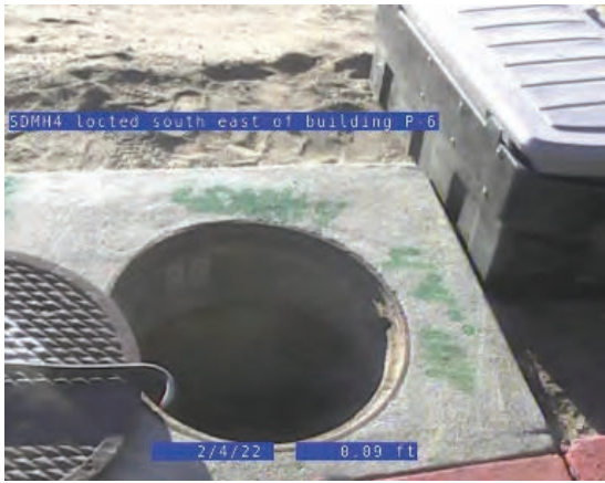
CCTV Entry Point Overview
