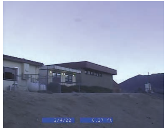
CCTV Entry Point Overall
