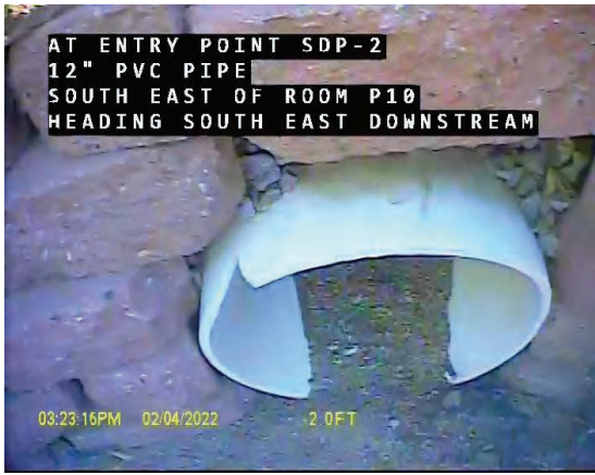
CCTV Entry Point Overview
