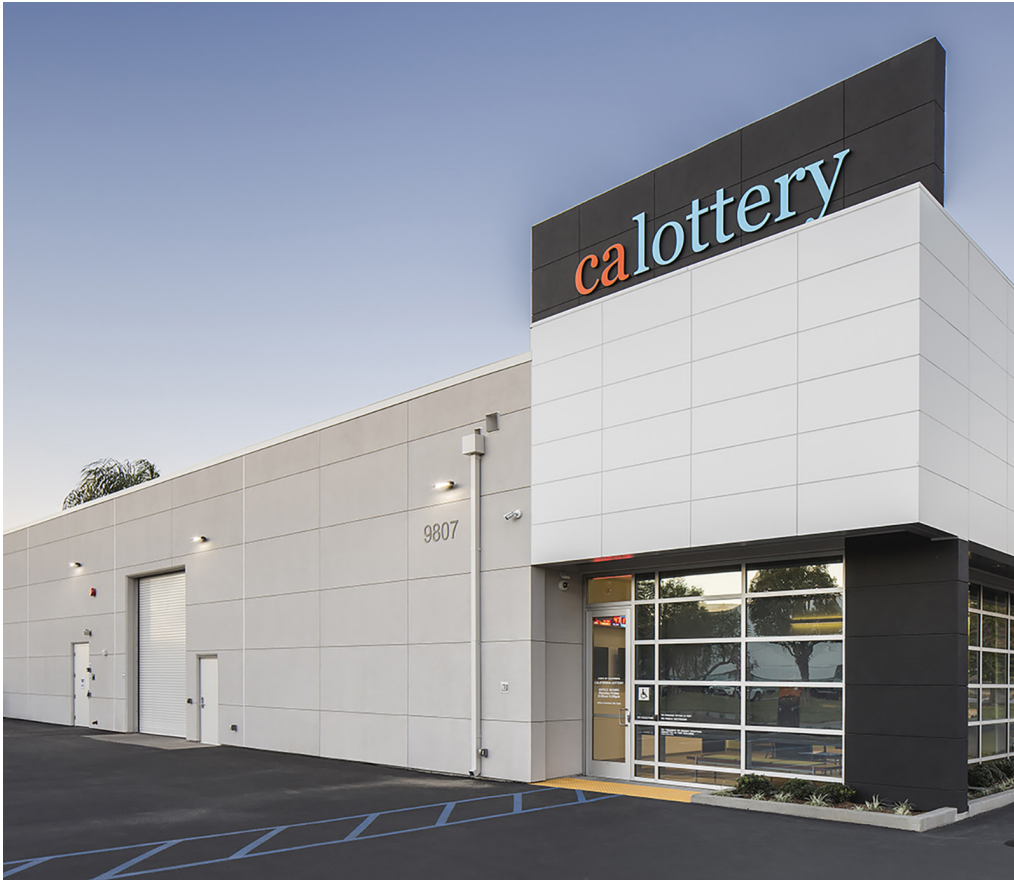
California Lottery Santa Fe Springs District Office.
