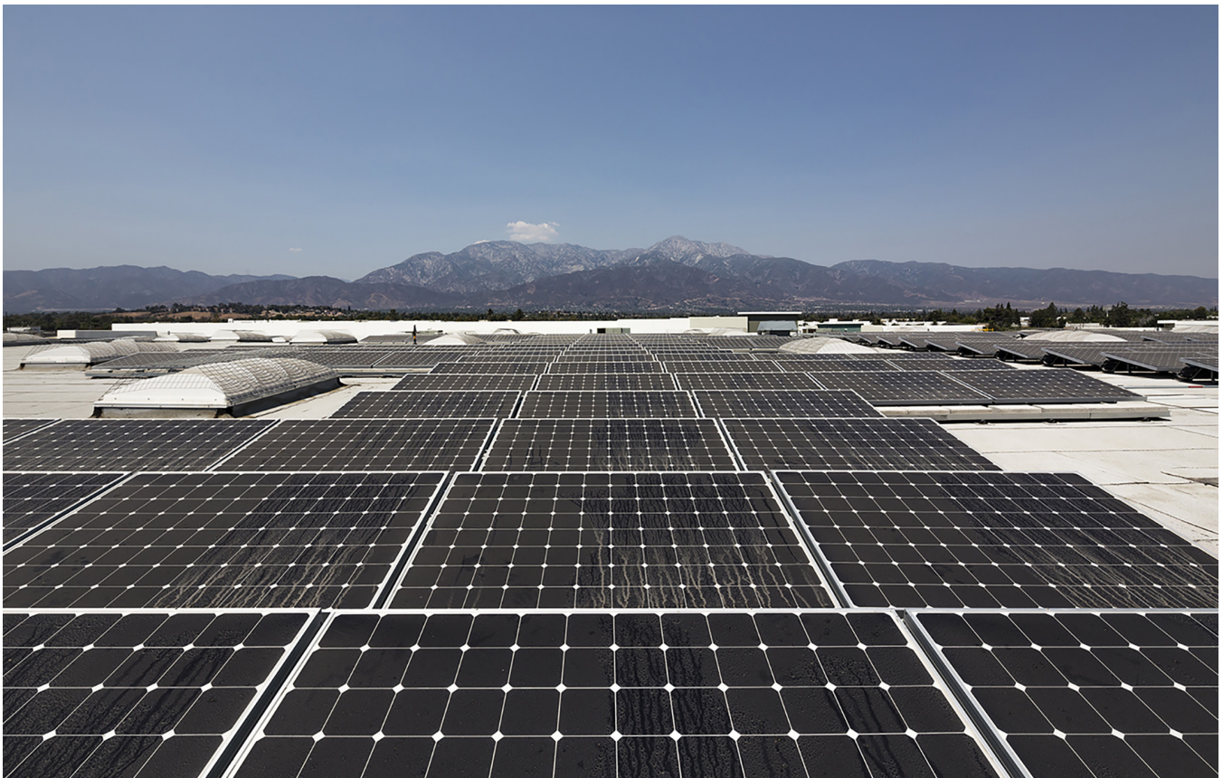
California Lottery Southern Distribution Center. Source: LPAS Arch + Design
